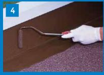
Apply the second layer of ALSAN FLASHING (700 g/m2).
