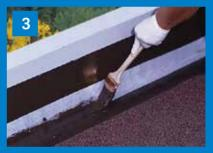
Apply the first layer of ALSAN FLASHING (900 g/m²).
