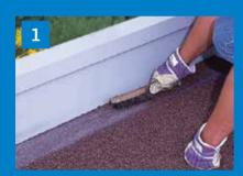
Remove all loose materials and granules from the area with a metallic brush. The area should be clean, dry and free of loose particles.
