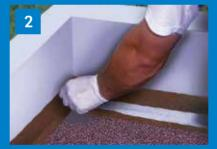
Apply a base coat of ALSAN FLASHING with a brush (500 g/m2) on the surface, lay FLASHING REINFORCEMENT and embed it in the base layer.
